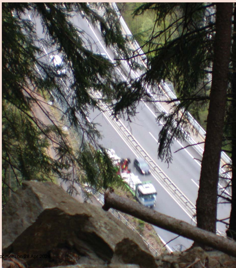
FIGURE 1 Rockfall threatens trans-Alpine transportation infrastructure. (Photo by J. Heeb)
