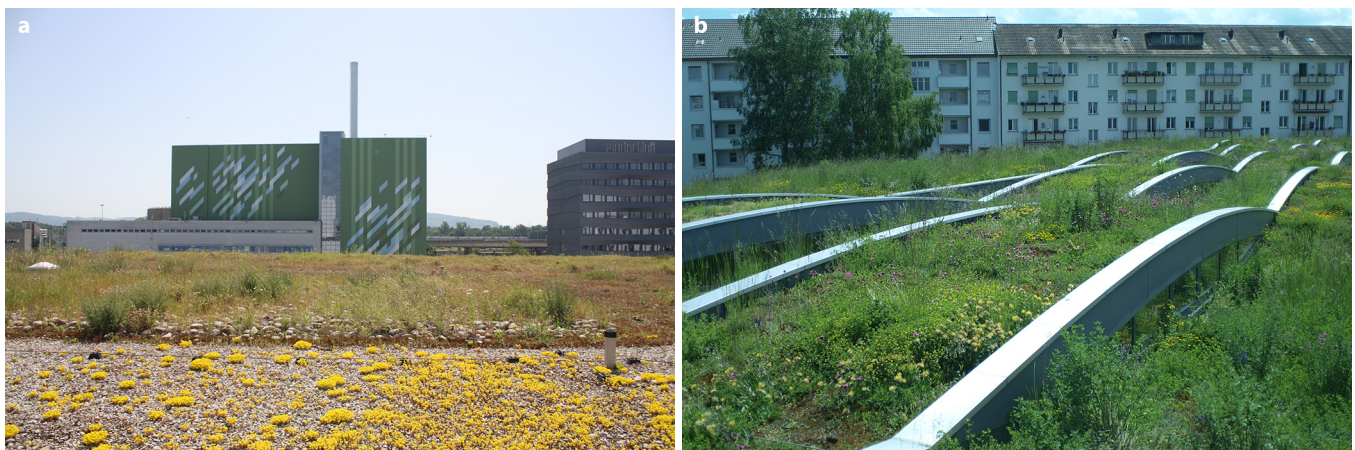
Fig. 8: Further habitat types on green roofs in Basel. a. Stücki Shopping Center, constructed to imitate some habitats on riverbanks; b. the green roof on the tram depot Wiesenplatz with higher vegetation density (Photos: Stephan Brenneisen)
