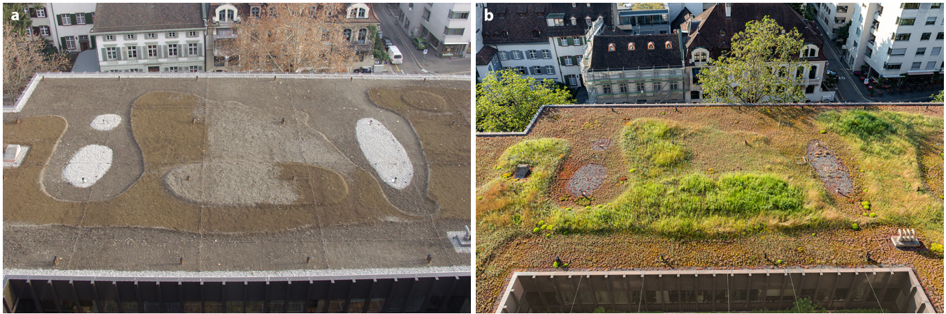
Fig. 1: Green roof of the University Hospital Basel, Klinikum 2. The pictures show a diverse substrate composition and varying thickness thereof. a. after installation in 2003 (Photo: Stephan Brenneisen); b. how vegetation composition is adapting to the different habitat conditions over the years. The picture was taken in 2021 (Photo: Andreas Hofstetter)
