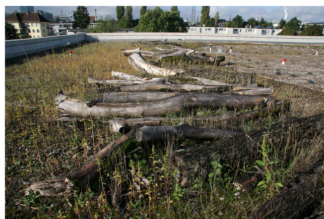
Fig. 7: School building Schoren, Basel, a green roof with a mixture of sandy gravel, compost, lava-pumice and wood, constructed in 2017. The site where Robertus mediterraneus was found for the first time north of the Alps (Photo: Stephan Brenneisen)
