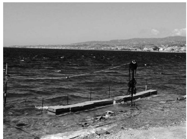
Figure 8. View of the vertical breakwater in shallow water used in the 2013 experiment.
