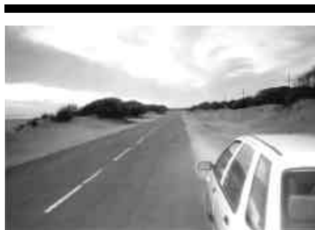
Figure 2. Existing road alongside La Bota beach (Huelva, Spain), Gómez-Pina 1997.
