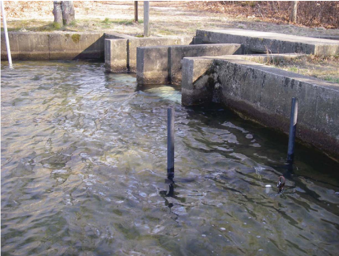
FIGURE 4. Photograph of study site 2 at the outlet of Hinckleys Pond. The DIDSON, attached to the black frame in the lower portion of the photograph, is aimed toward the opening of the fishway.
