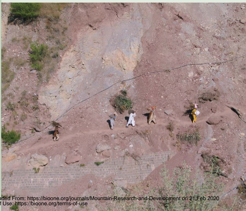
FIGURE 1 Critical infrastructure was impacted by landslides after the earthquake, forcing people to improvise in order to survive. (Photo by J.P. Hamilton, November 2005)
