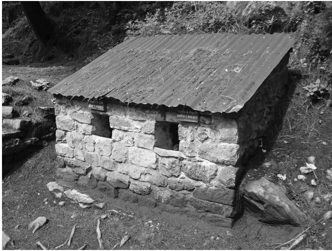
FIGURE 6 One of the approximately 70 litter bins installed by the SPCC throughout the national park and buffer zone. (Photo by Alton C. Byers)
