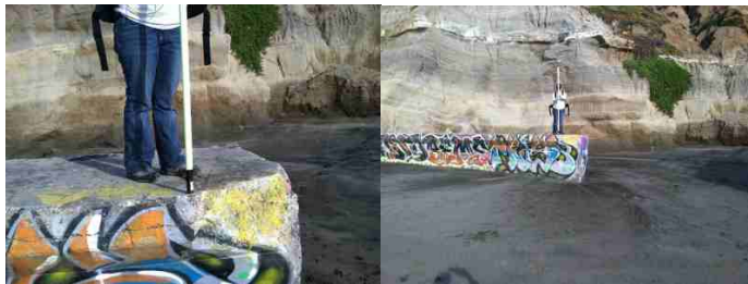
Ground Control Point 123: Corner of northern outlet structure at base of cliffs.
