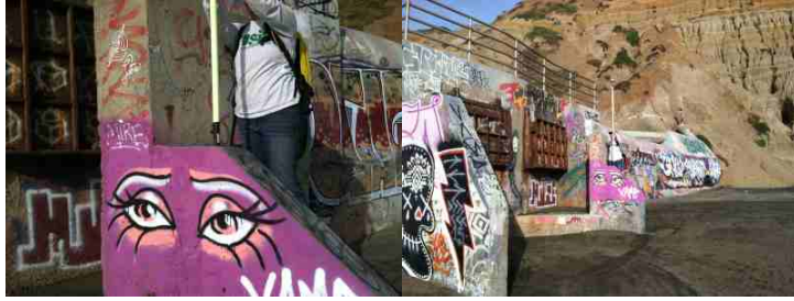
Ground Control Point 125: Corner on southernmost end of the southern outlet structure at base of cliffs.
