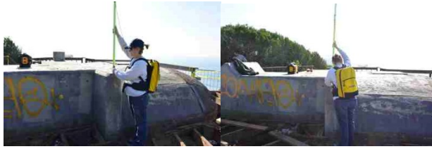
Ground Control Point 13: Northern corner of southernmost small battery in the “Funston Group”
