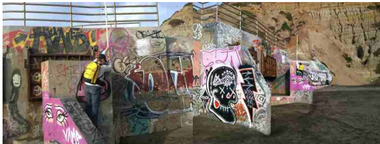
Ground Control Point 126: Corner on southernmost end of the southern outlet structure at base of cliffs.
